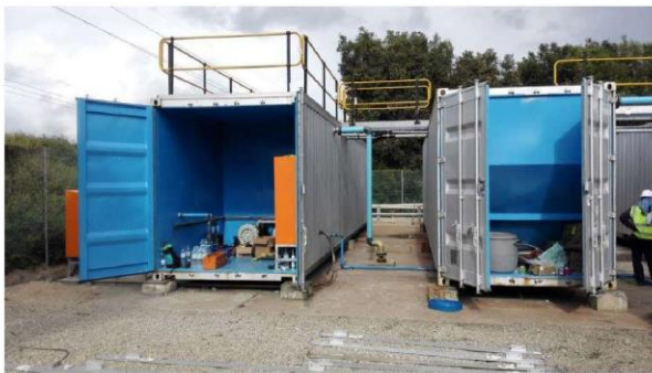
180m 3 /day Containerised Sewage Treatment Plant - Madagascar
