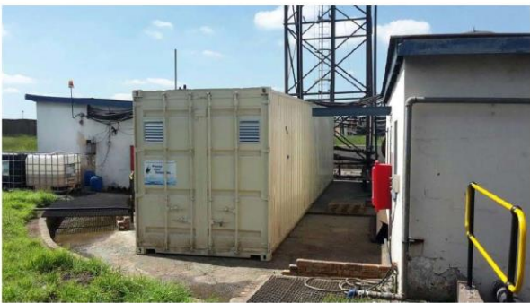
25m 3 /hr Containerised Reverse Osmosis Plant - South Africa
