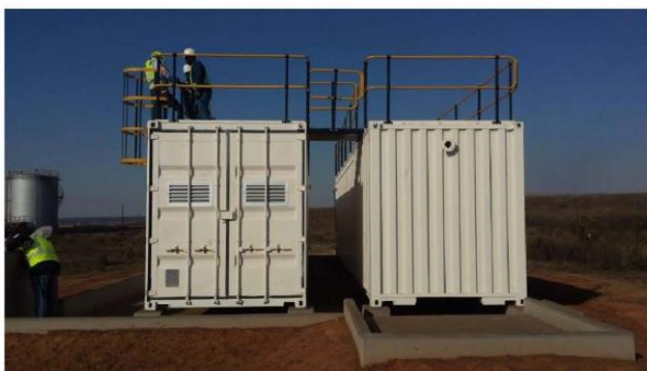
80m 3 /day Containerised Sewage Treatment Plant - South Africa
