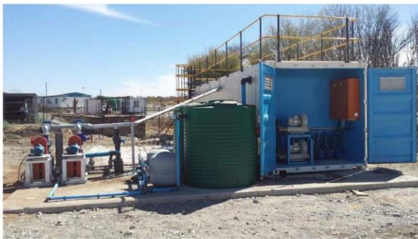
40m 3 /day Containerised Sewage Treatment Plant - South Africa
