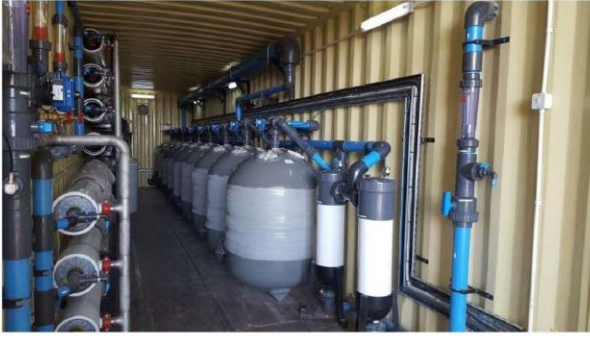
30m 3 /hr Containerised Reverse Osmosis Plant - South Africa
