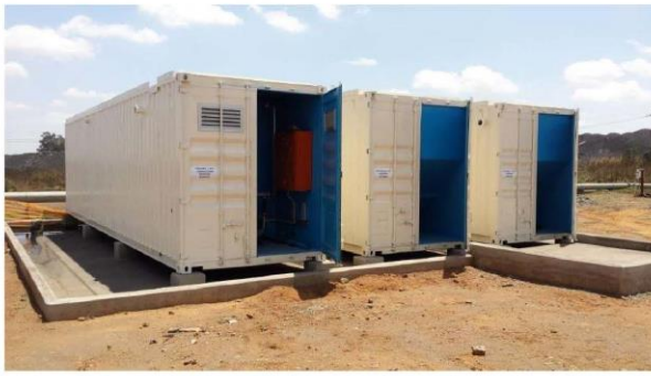
135m 3 /day Containerised Sewage Treatment Plant - South Africa
